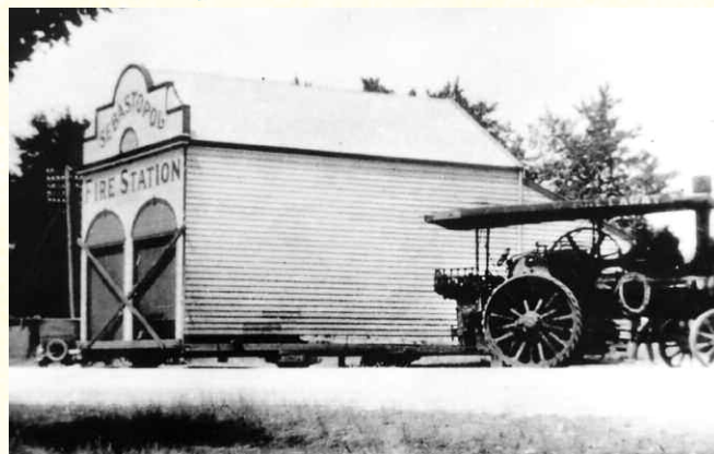
Nunn's traction engine assists in the removal and resiting of the fire station. (Source: Nunn Bros Haulage, 31 Wiltshire Lane, Ballarat)
