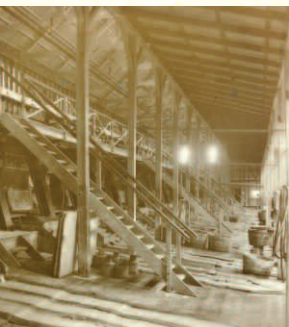
Battery house, Star of the East, Ballarat, J.H. Harvey, photographer, [between 1875 and 1938], lantern slide. (Source: State Library of Victoria)
